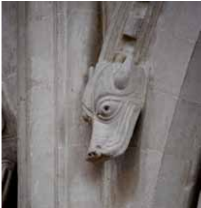
Malmesbury Abbey Nave. Animal head completes the hoodmould above an arch in the arcade
